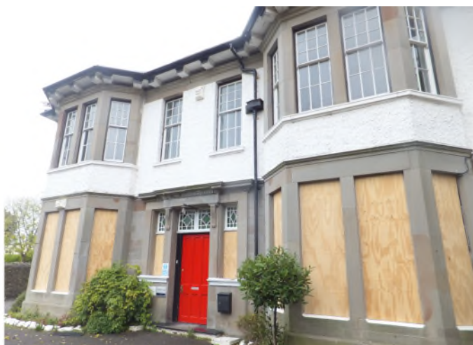
Fig. 1 - Photograph of Existing Rectory Building
